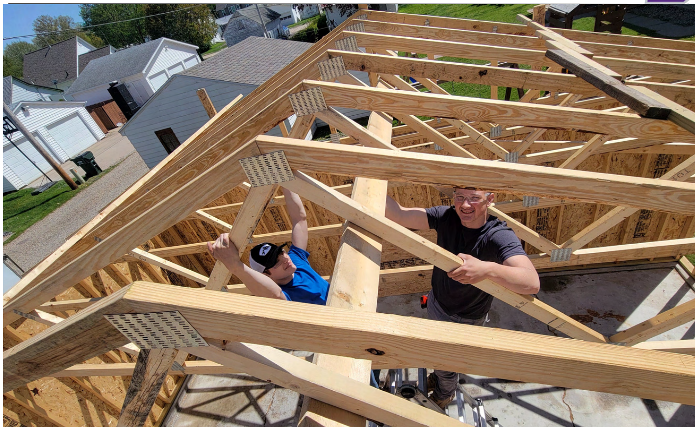
Students in Kyle Krieger’s Construction Trades class work on a three-car garage for an area resident. They started the project this past spring and completed it Nov. 1.
